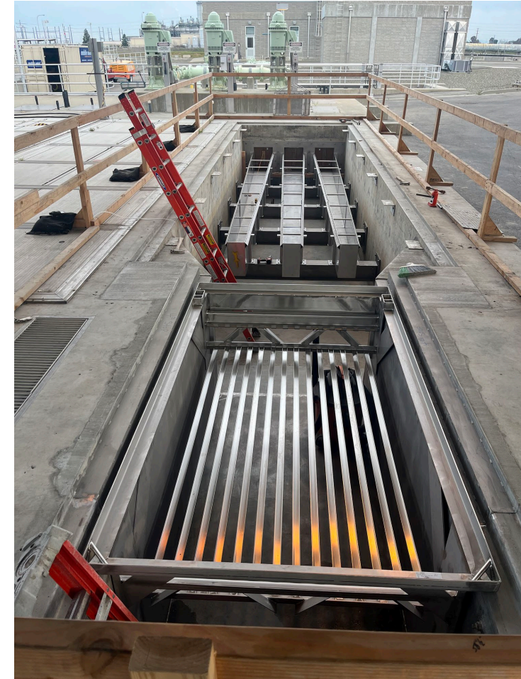
Adding new light bank and weirs
